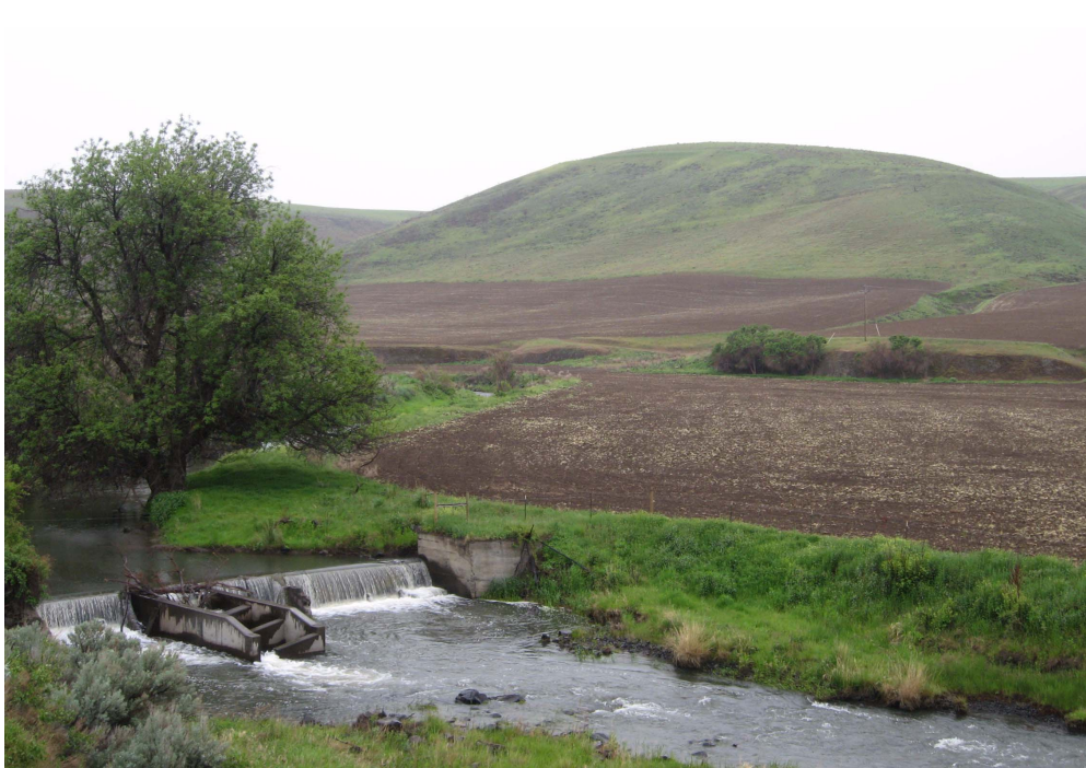
Figure 9.5. Fish ladder on a concrete irrigation dam located on the mainstem of Rock Creek, Gilliam County, Oregon.
