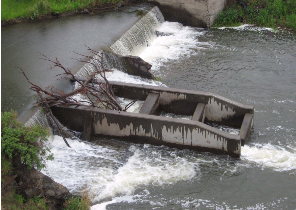
Figure 11.8. Bettencourt Diversion on mainstem Rock Creek with fish ladder installed by ODFW in 2005, Juniper Canyon subwatershed, Oregon.
