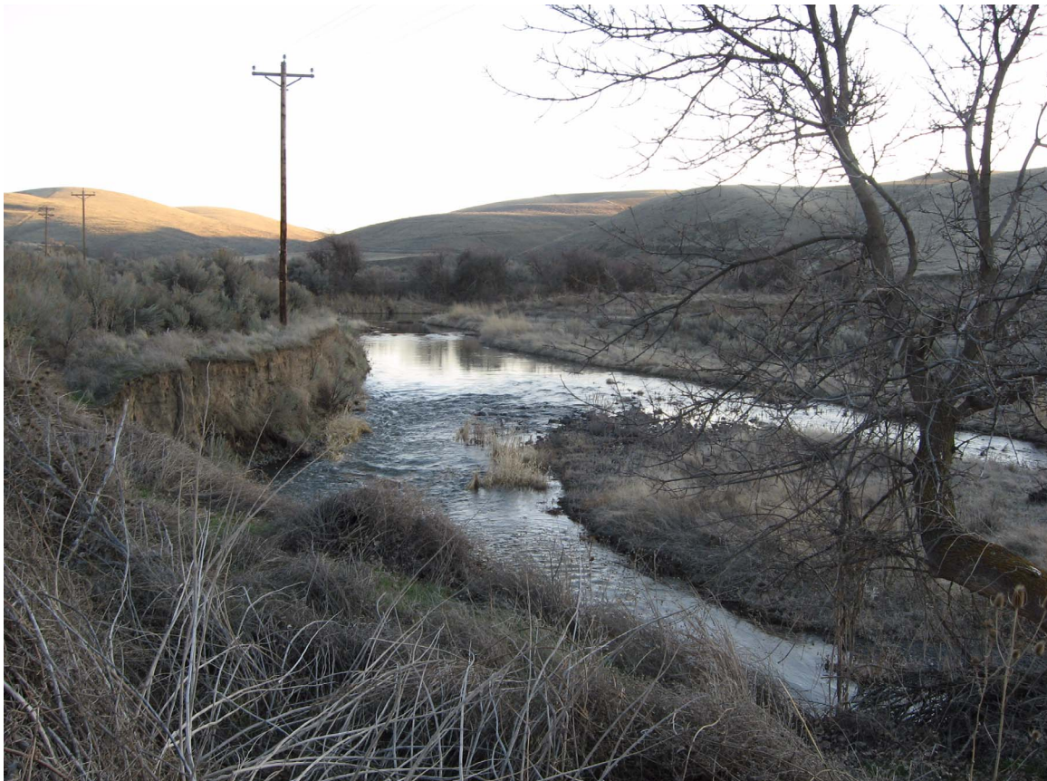
Figure 8.11. Example of a section of Rock Creek with severe bank erosion.
